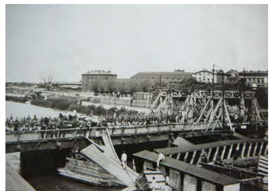
The pool was destroyed by the river and it got stuck by the bridge.
